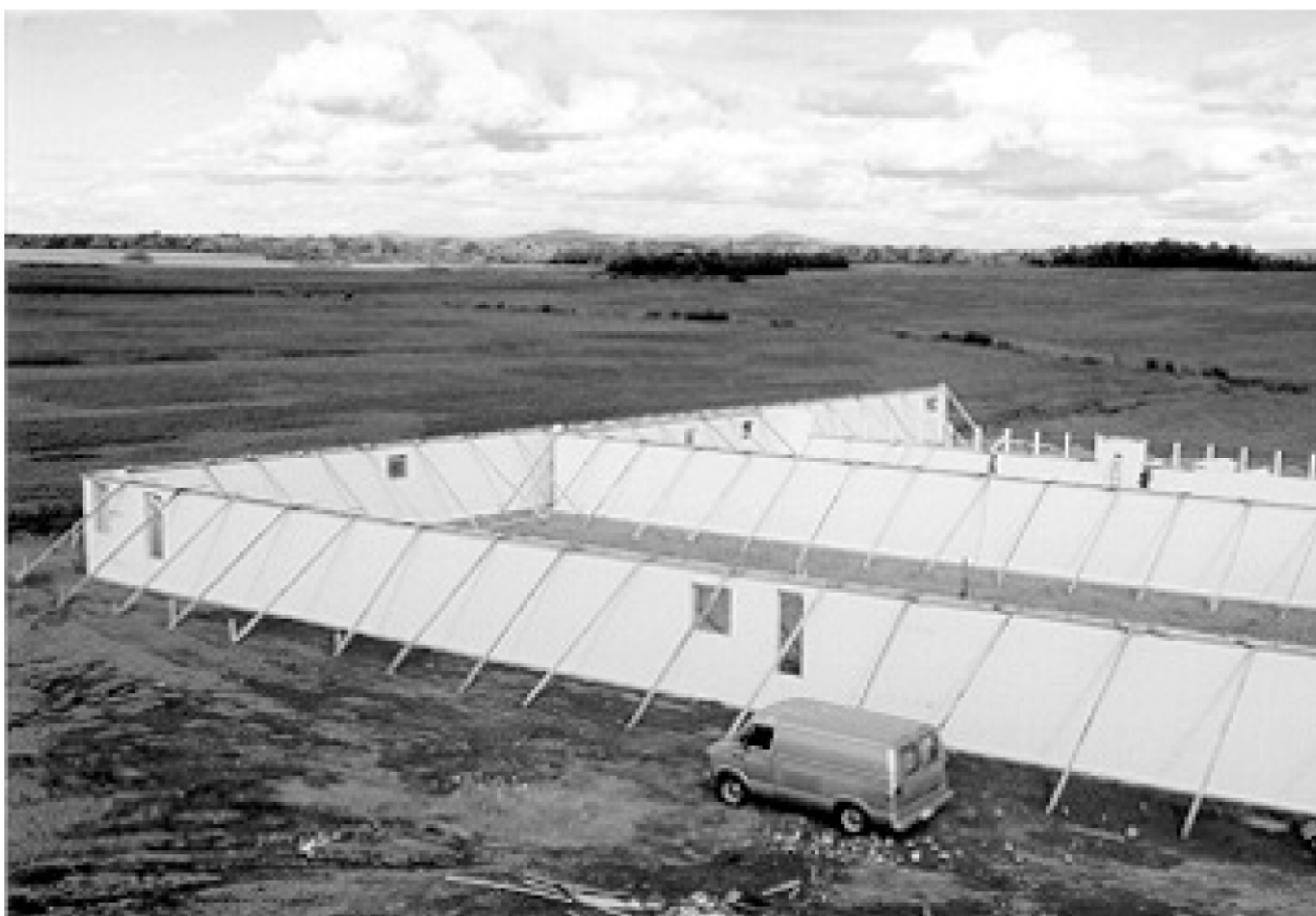
2.2 Bearing Wall Project in Progress
