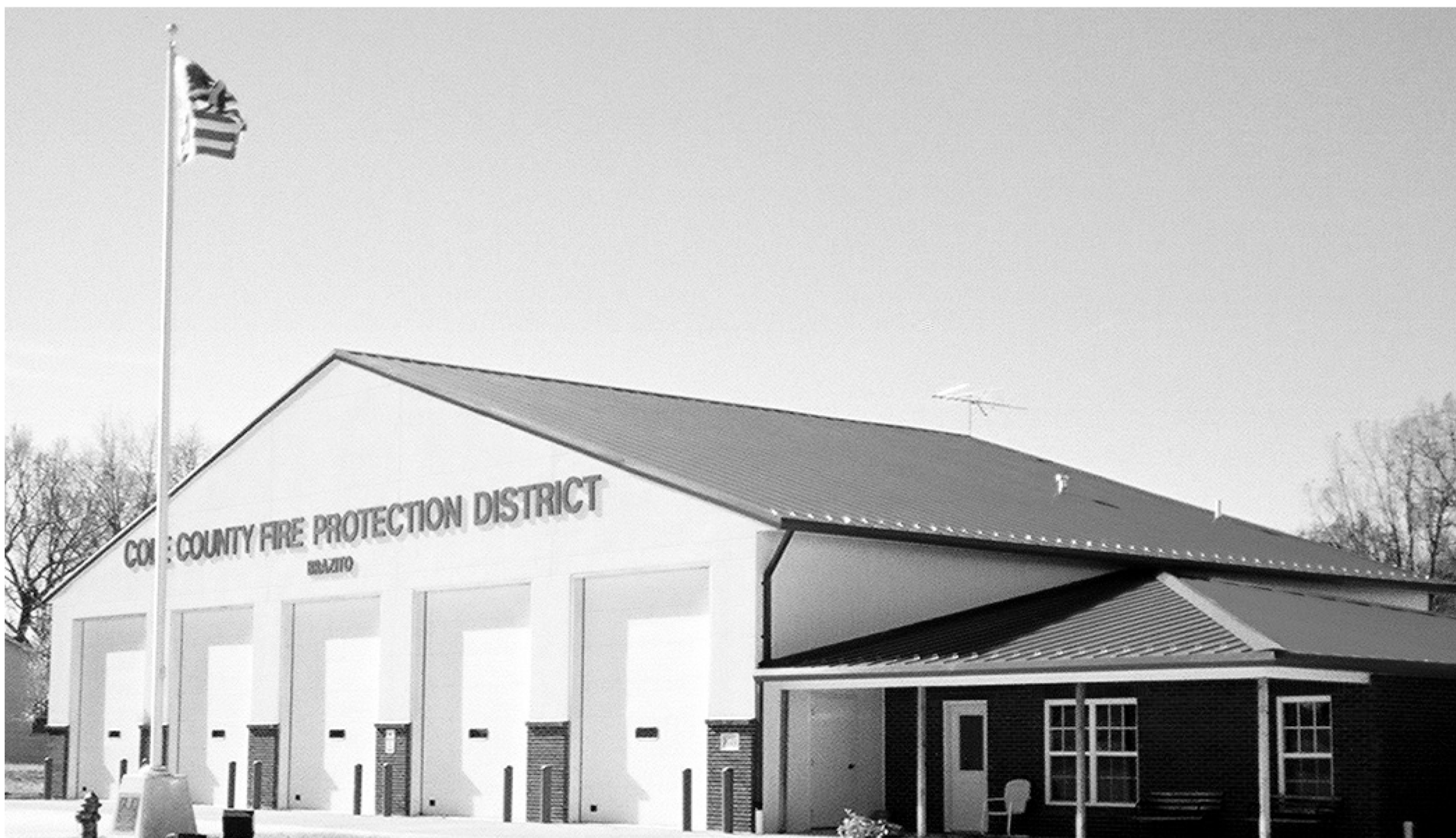
1.0 Bearing Wall Project
