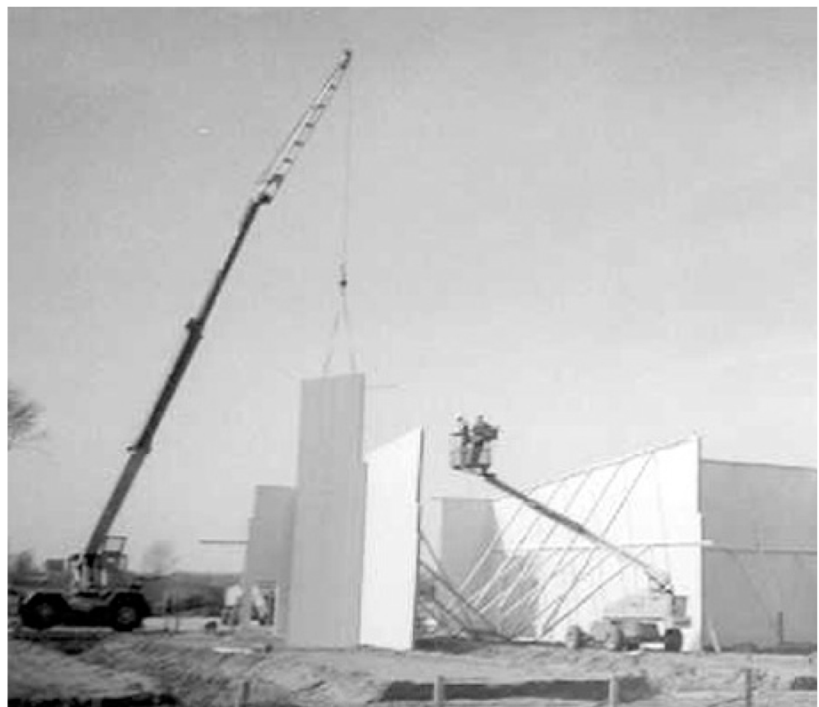
2.4b Erection of Pre-assembled Wall Section
