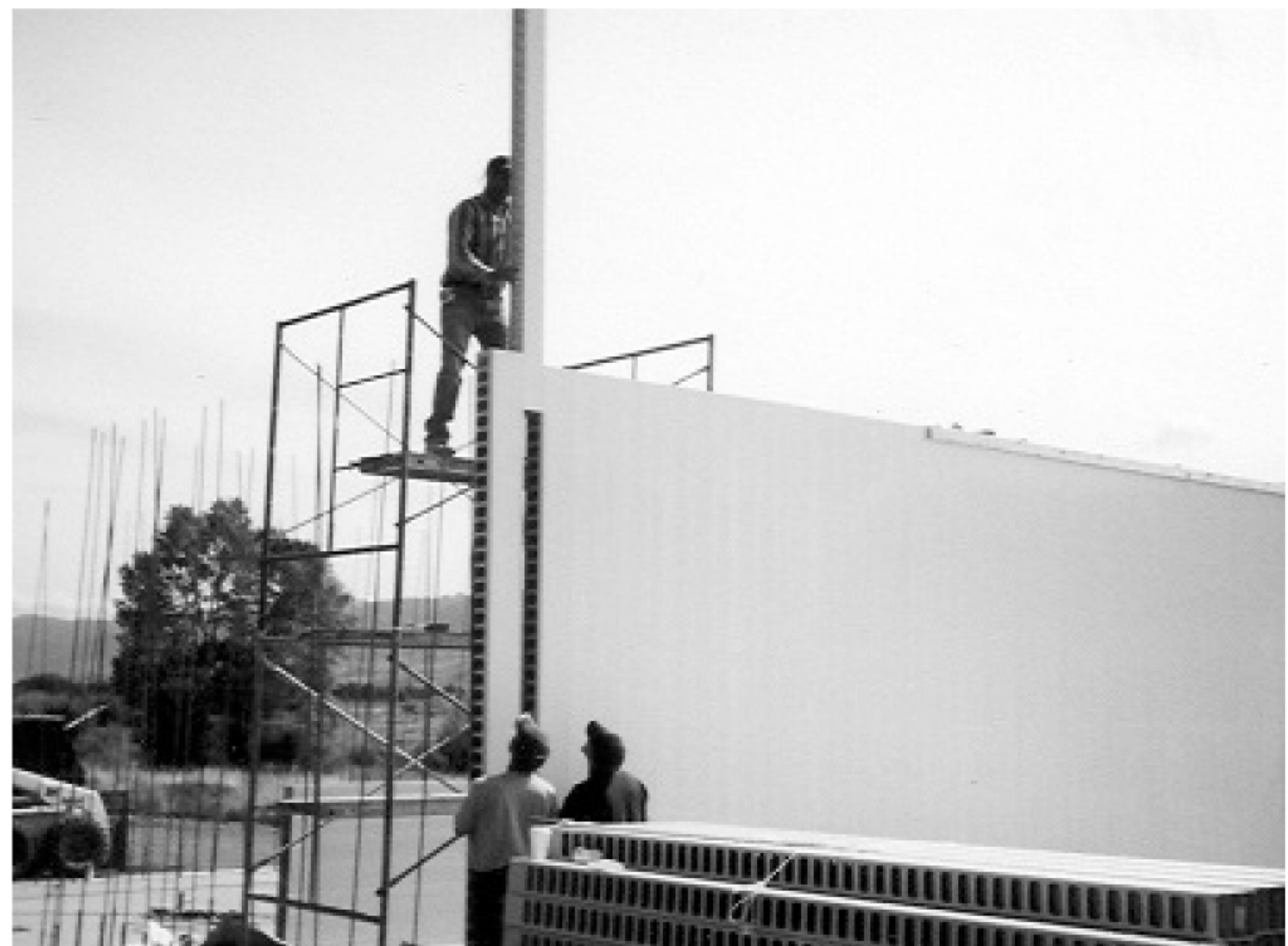
2.3 Construction using Individual Components
